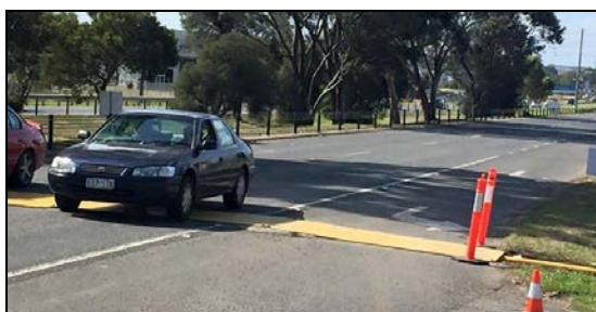
The large yellow 100mm hose provides water from different sources
