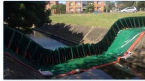
Pictured: The Rapidam in action.
