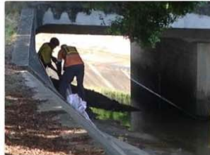
Pictured: Ben Patterson (RHDHV) and Justin Bear (Bluemont) filling sandbags.
