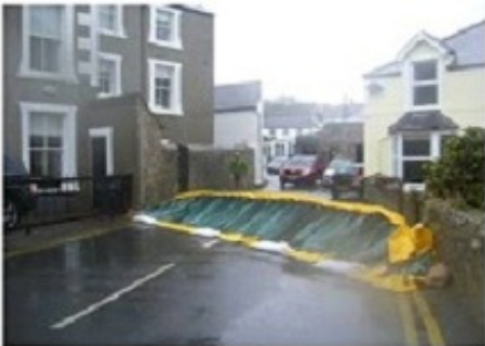
Alteau flood barrier in place
